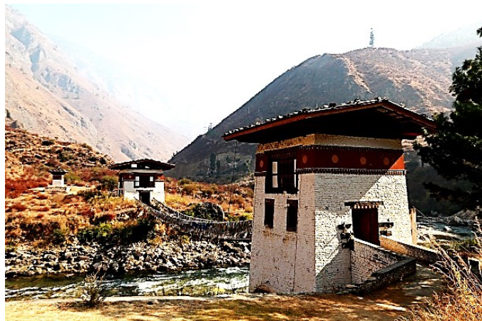
Fig. 69: a historical suspension bridge with iron chains. Tamchog Chakzam (XV th c.)
