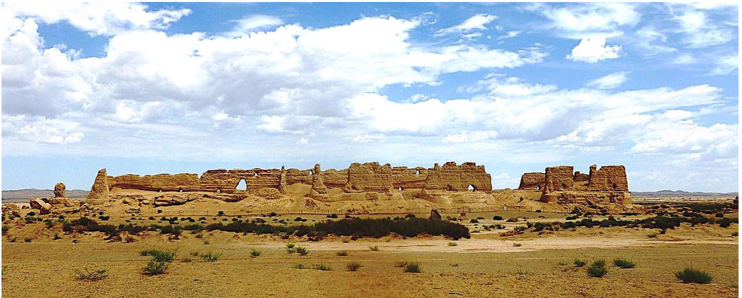
Figure 7: ruins of a granary in the fortress of Hecang near the Yumen pass, 75km north-east of Dunhuang (Western Han, rebuilt during the Western Jin period around AD 280-316). Evident strategic role of grain
